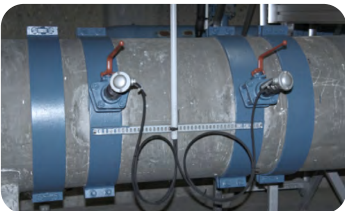
Flow measurement of water intake – Méry-sur-Oise water treatment plant – France
