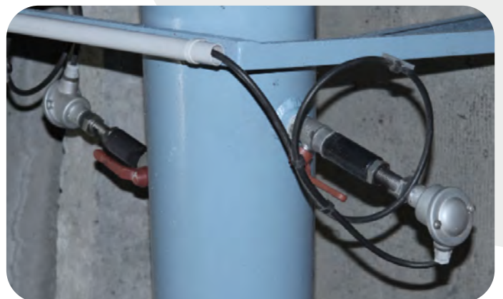
Flow measurement of water intake – Méry-sur-Oise water treatment plant – France
